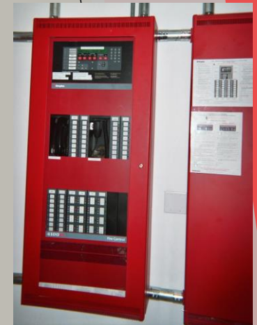
FIRE ALARM PANEL IN Fire Command Center (FCC)
